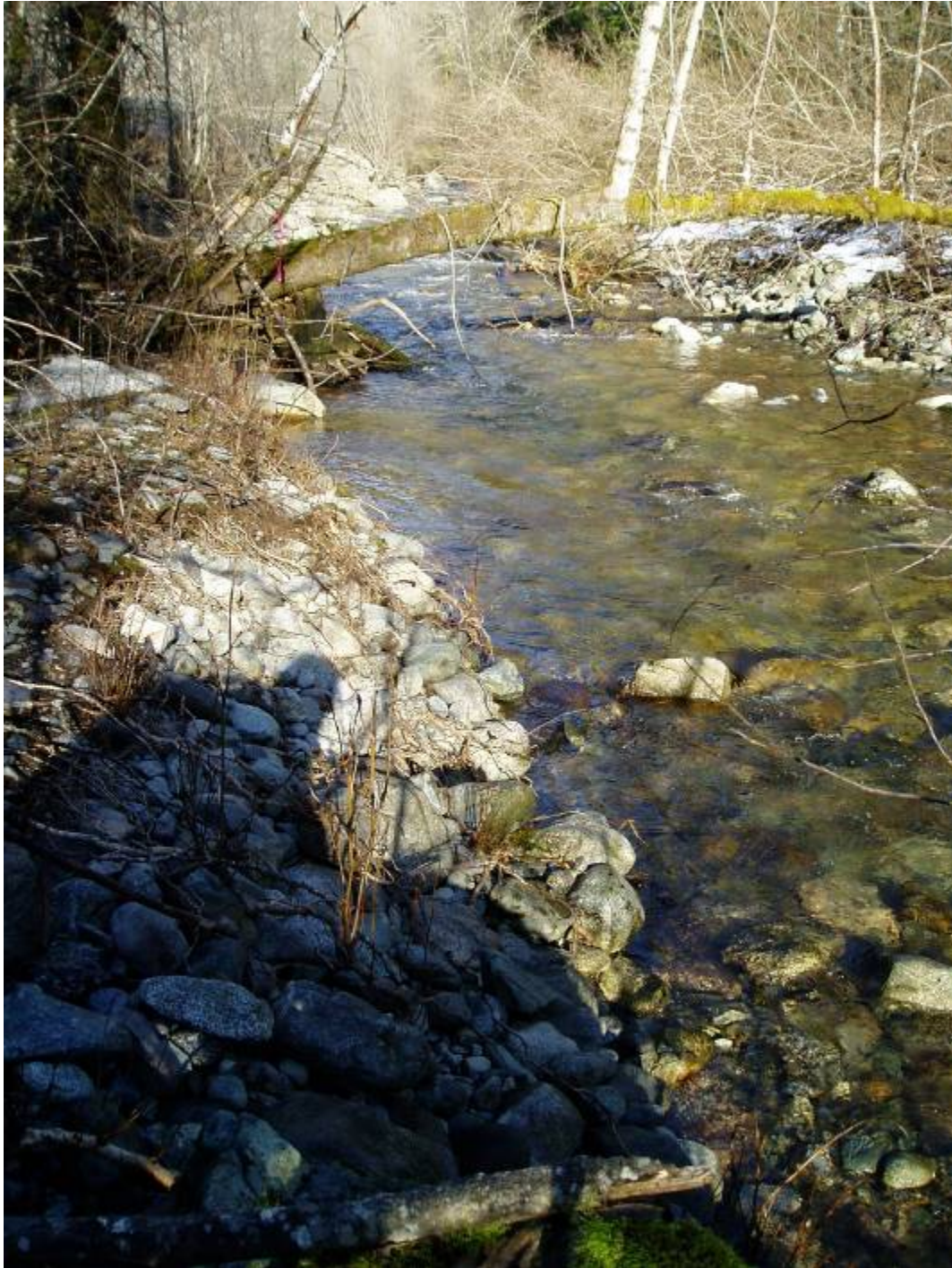
Appendix Figure 12. Reach-2 1218 m riffle: 2-rootwad 0-ramp right bank flat triangle (under overhanging cottonwood), plus 12 3-boulder within tail-out (2-3 clusters) and within highway-encroached steep riffle upstream (9-10 clusters), within thalweg with boulders 0.5 m apart and clusters 3 m apart.
