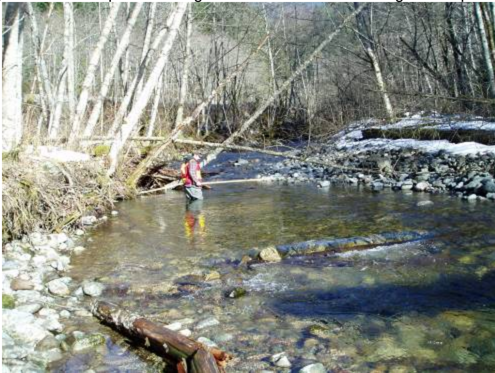
Appendix Figure 8. Reach-2 921 m glide-run: 2-rootwad 2-ramp log right bank triangle for prime rearing/wintering habitat and potential sp. gravel deposition.
