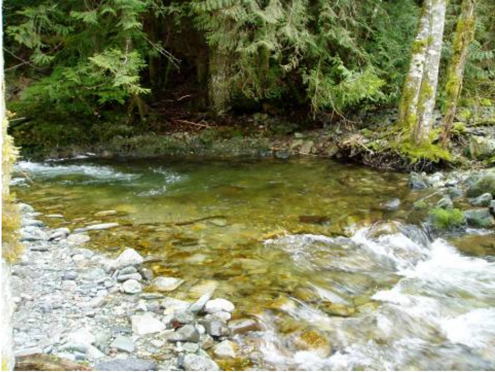
Appendix Figure 20. Reach-6 3049 m glide-run; Newbury riffle using local 0.3 m to 0.6 m boulders to augment spawning gravel deposition (local boulders reliant).
