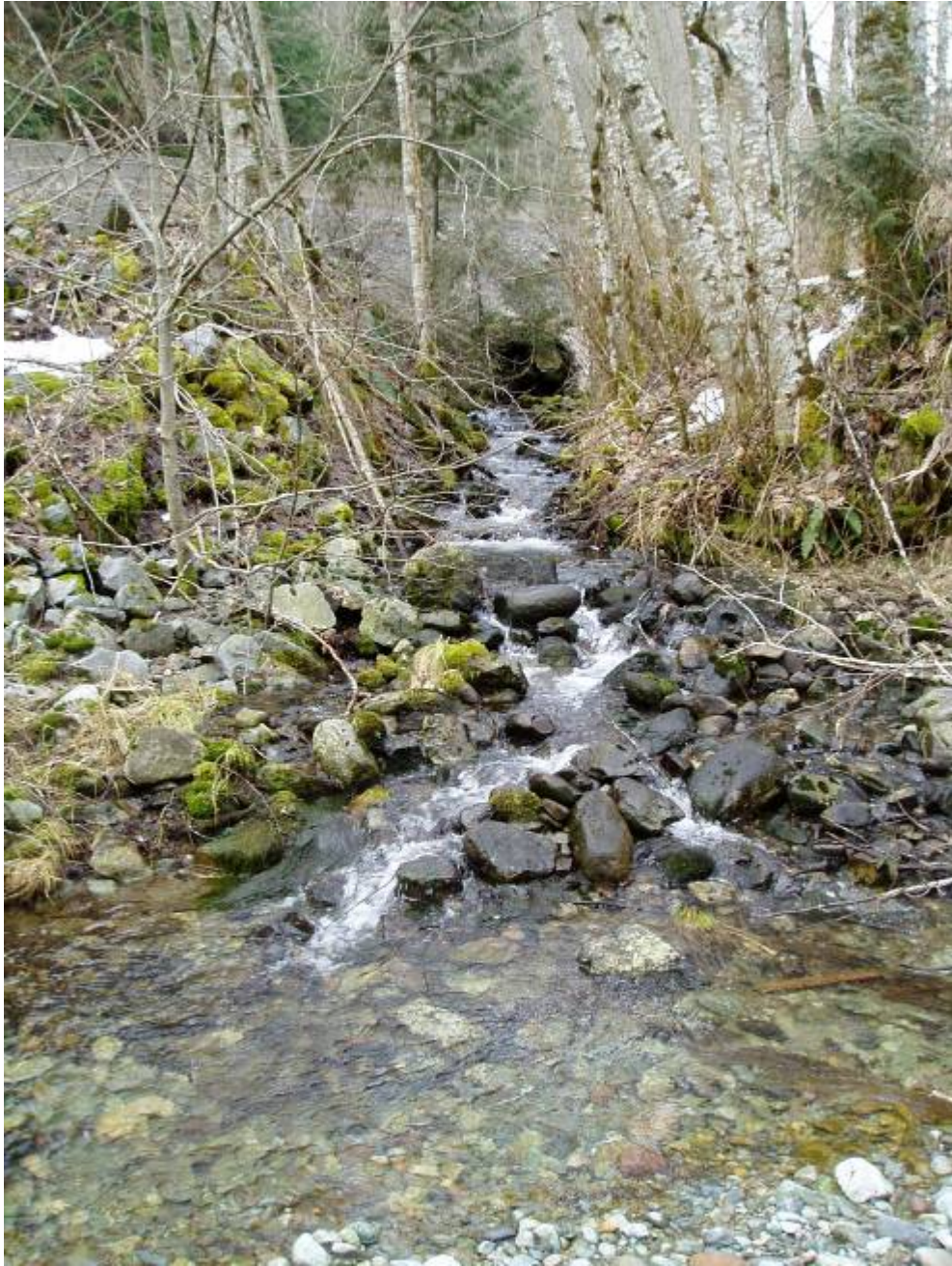
Appendix Figure 17. Reach-2 1600 m highway-culverted west tributary: Newbury riffle to elevate residual depth to backwater culvert for access of coho spawners at moderate to higher fall flows, with later baffle installations. (Note: subject to hydraulic engineering input and MoT approval)
